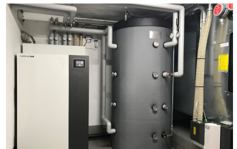
Pellet boiler (left) and buffer tank in a two family building. Photo: Bea Heitzmann
