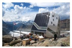
An impressive 122 m<sup>2</sup> photovoltaic cell installation on the south side of the hut together with a new combined heat and power (CHP) plant provides electricity for waste water treatment, ventilation, lighting and household appliances.
