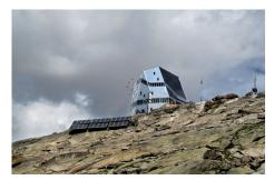
In front of the hut 60.5 m2 of thermal solar collectors have been installed. These cover the thermal requirements for heating and hot water preparation in combination with the CHP plant.
