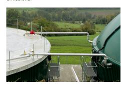
A double-membrane roof on the fermentation tank and a covered final repository for fermentation residue ensure that no methane escapes into the atmosphere (Foto: Klimastiftung Schweiz).
