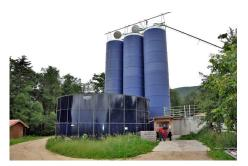
After fermentation, nutrient-rich fermentation slurry is held in the final repository and later applied to fields as fertilizer. Foto: myclimate
