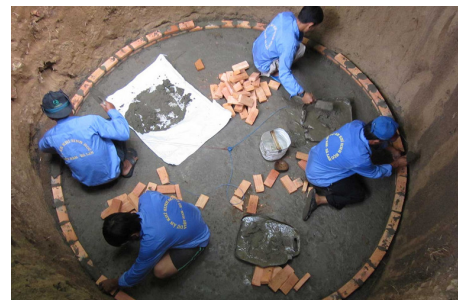
Construction of a biodigester with bricks and clay. Photo: Nexus for Development
