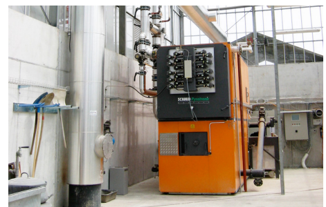
1'600 kilowatts wood heating system in a greenhouse at BioLand Agrarprodukte in Steinmaur ZH. Photo: Daniel Meier
