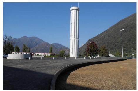
The chimney above the underground wood chip heating plant The heating plant provides the school building (red building in background) and other buildings with heat from renewable energy.
