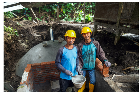
Nathun and his son are working on the construction of a fixed dome in the construction of a biogas installation. Photo: Gema Ramadhan
