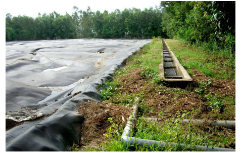
A membrane captures the climate-damaging methane gas.
