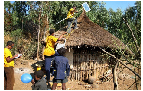
Installation of a Solar Home System in the village.
