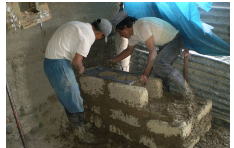
Local artisans building a new stove with chimney.
