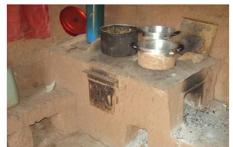
The newly-installed chimney (blue pipe to the left) leads the smoke out of the house.
