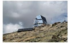
In front of the hut 60.5 m2 of thermal solar collectors have been installed. These cover the thermal requirements for heating and hot water preparation in combination with the CHP plant.
