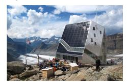
An impressive 122 m² photovoltaic cell installation on the south side of the hut together with a new combined heat and power (CHP) plant provides electricity for waste water treatment, ventilation, lighting and household appliances.
