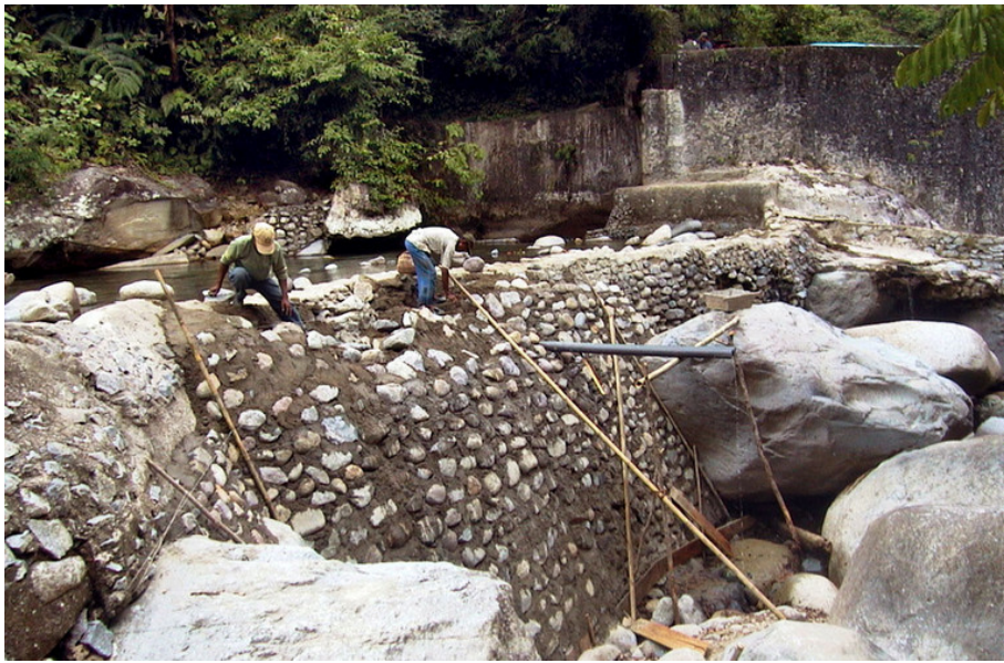
Reconstructing of the historical dam with local raw materials.
