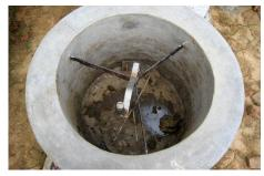
This crank is used for mixing the manure with water before it drains off in the plant.
