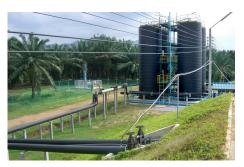
The methane gas is transferred to the gas cleaning system through the connecting pipes and is then burnt in the generator. This renewable electricity is used in the plant and fed into the grid.
